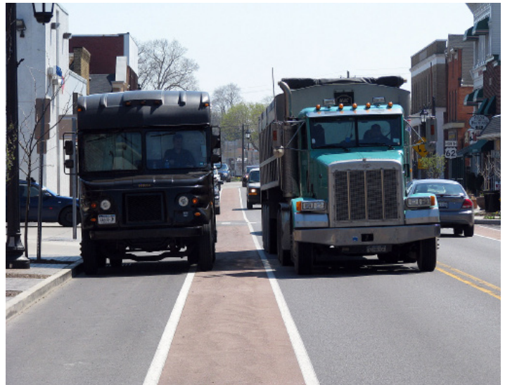
▲ Route 62, Hamburg, NY vehicle lanes are made narrower (10 ft) and a colorized “door-zone” buffer helps separate moving vehicles from people exiting/entering a parked car. Route 62 is a major truck route for the State of New York.
